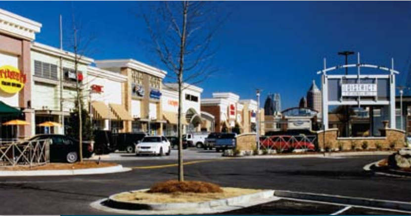
The District at Howell Mill Phillips Partnership, Atlanta, Ga.
